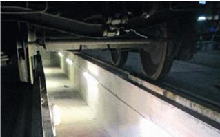
Covering the pits helps to secure the area by preventing falls into the pits when they are not in use
